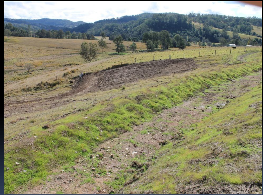
Construction of 2 roll-overs
